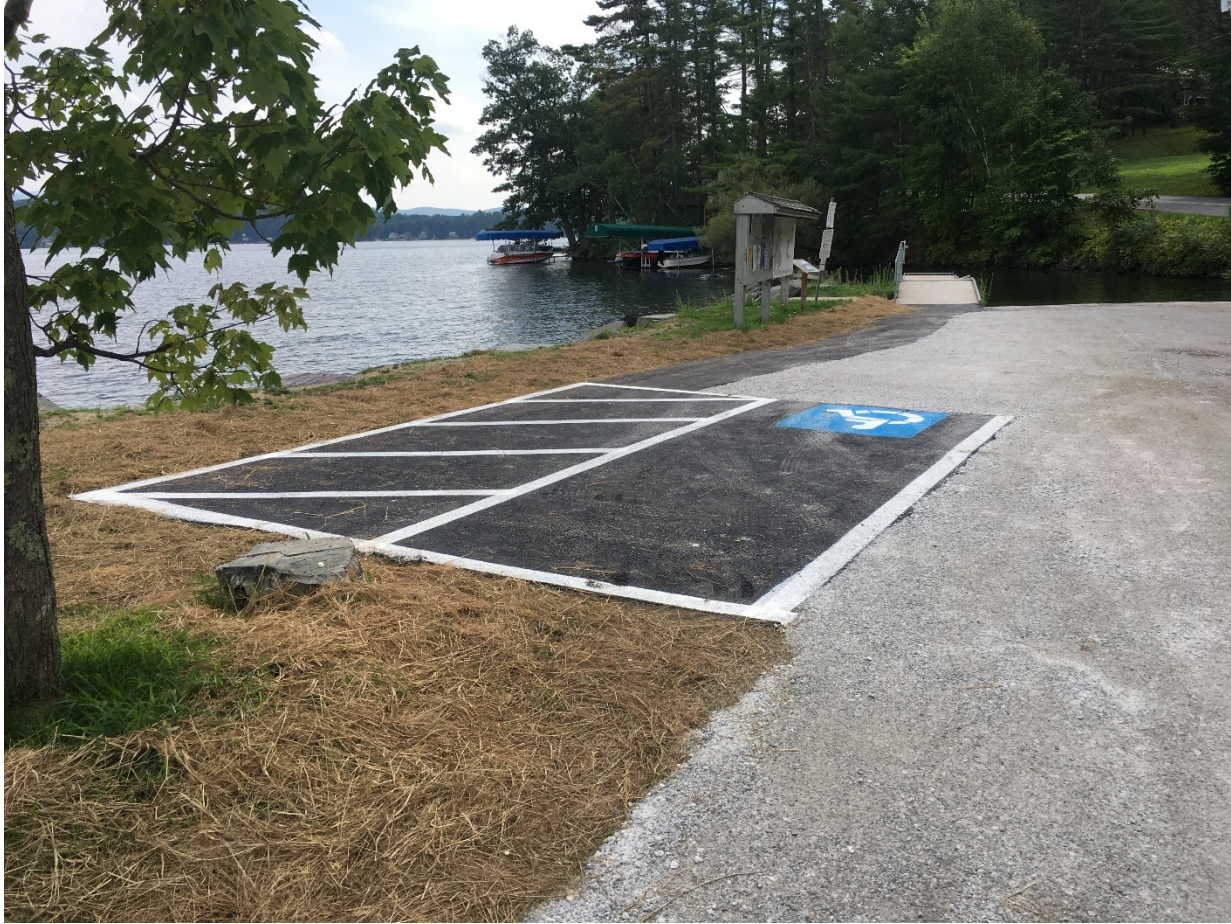
Figure 1. New ADA parking space constructed in 2018 and a new dock constructed in 2013 at the Kehoe Access Area, Castleton, VT.
