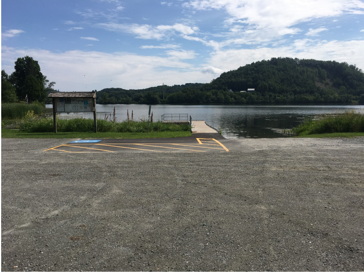
Figure 2. New ADA parking space constructed in 2018 and a new dock constructed in 2017 at the South Bay Access Area, Newport City, VT.
